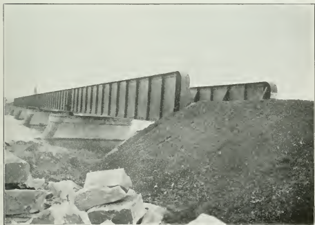
Intercolonial Railway, Riviere du Loup Subdivision. Bridge over River St. Nicolas.
