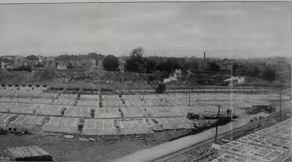
N. S. View of Shell Yard looking West from Mixing Plant.
