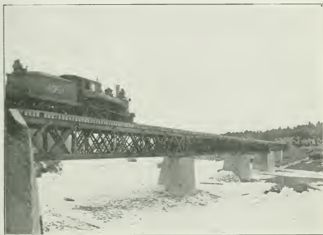
Intercolonial Railway. Nashuaak Bridge. Mile 105'3. Fredericton Subdivision. New steel bridge on concrete piers and abutments.
