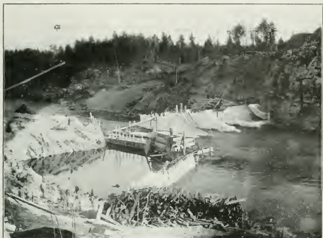
Trent Canal. Severn division. Bottom of Swift Rapids dam and wheelpit of power house.
