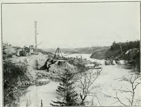
Trent Canal, Severn Division. Looking up the Severn River from below Swift Rapids.
