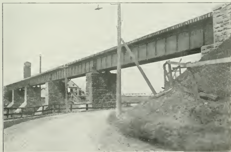
Intercolonial Railway, Mont Joli Subdivision. Bridge over Remouski River.
