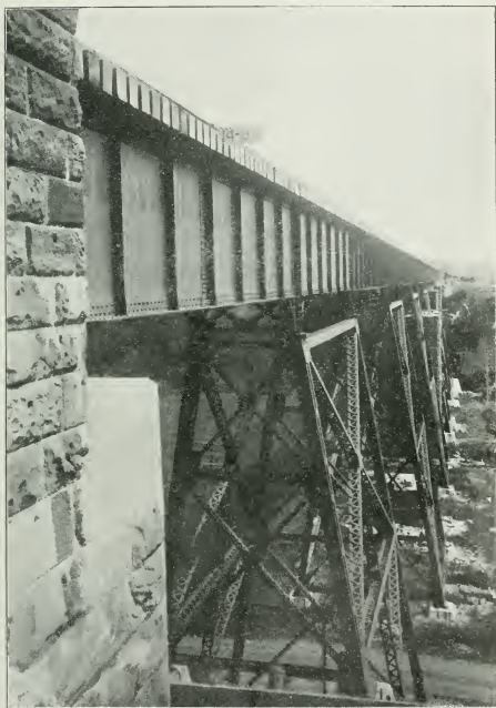
Intercolonial Railway, Truro Subdivision. Folliegh River Bridge.
