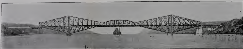
Quebec Bridge, across River St. Lawrence above Quebec, in course of construction.
