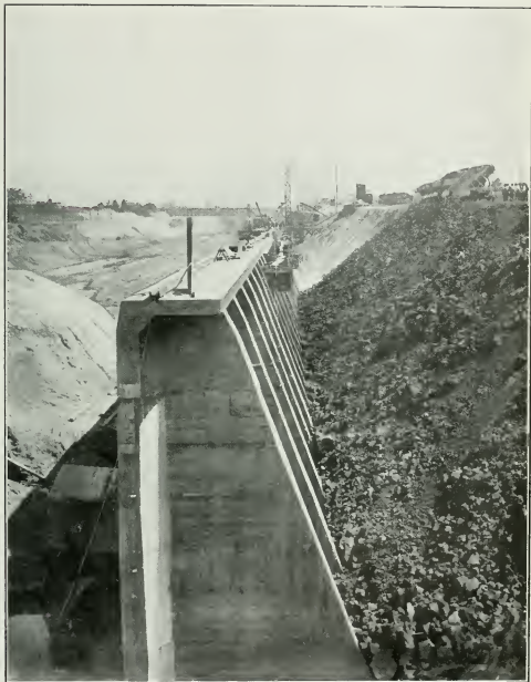
Welland Ship Canal. Reinforced concrete Entrance Wall, Lock No. 1, being backfilled.
