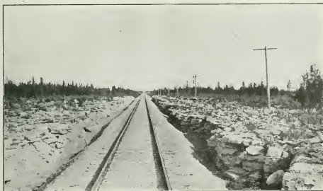
Hudson Bay Railway. Cut at Mile 53 looking north.
