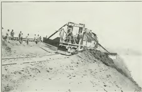
Welland Ship Canal. Spreader at work on Harbour Embankment.
