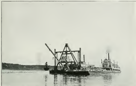
Hudson Bay Railway Terminus, Port Nelson. Excavating boulders, for crib filling and riprap, from river bed near Flamborough Head. The orangepeel dredge, scows and stern wheel tug, in rear, were built at Port Nelson.
