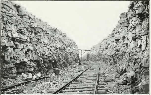
New Welland Ship Canal. Rock cutting for diversion of Grand Trunk Railway, Thorold.
