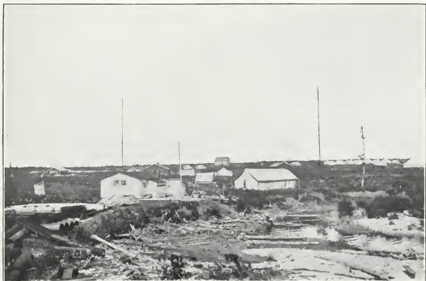
Hudson Bay Railway. Eastern end of encampment, showing wireless installation in background.
