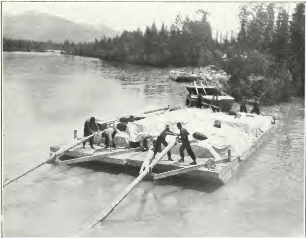
Grand Trunk Pacific Railway. Contractors' supplies scows on the Fraser river at Tête Jaune Cache, B.C.
