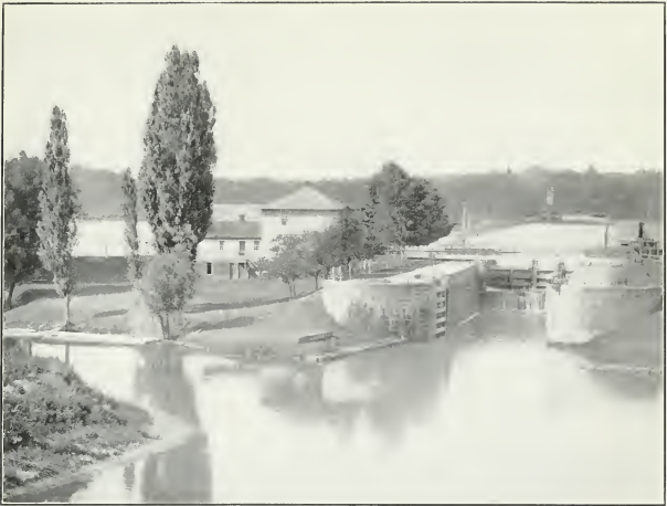
Rideau Canal. Washburn Lock.
