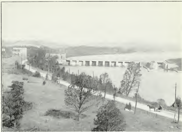
Trent Canal. Lock and Dam No. 2, at Trenton.
