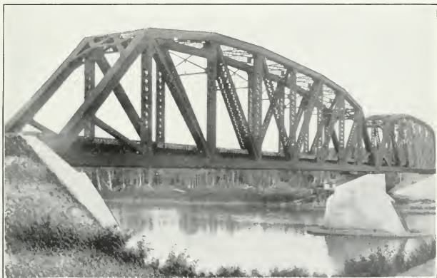
Transcontinental Railway. Bridge over the Ground Hog River, 1,078 miles from Moncton.
