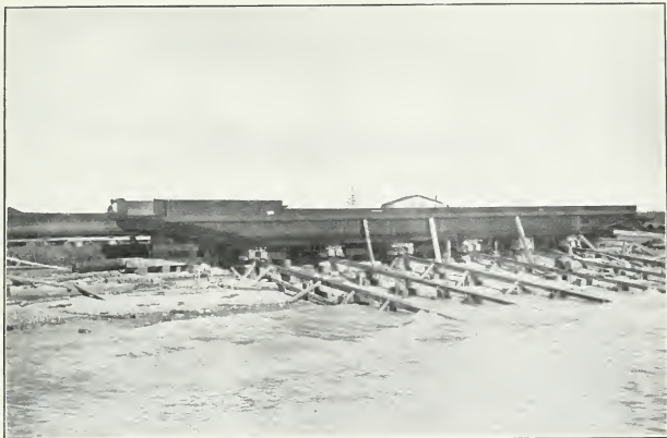
Hudson Bay Railway. Hull of stern wheel tug assembled and ready for launching.
