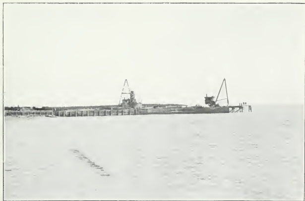
Hudson Bay Railway. Wharf No. 3, Port Nelson.
