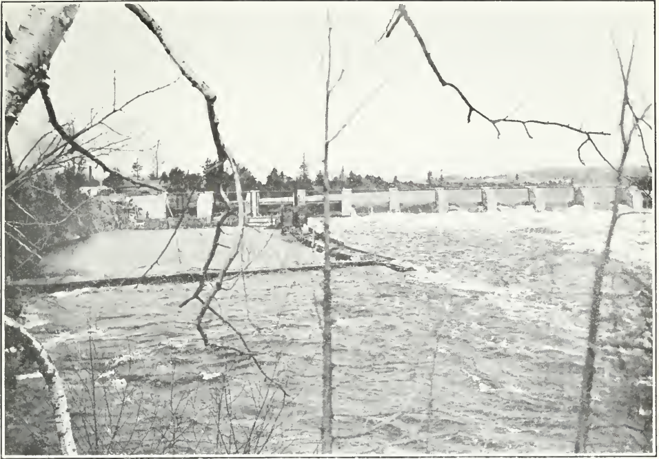
Trent Canal, Ontario—Rice Lake division dam 5, with coffer dam for power house.
