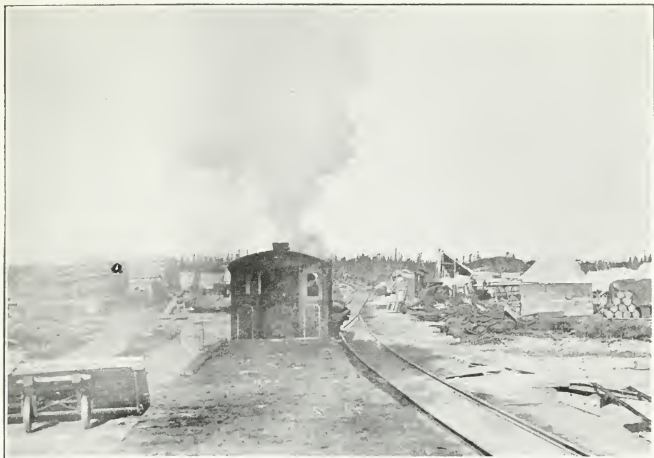
Hudson Bay Railway—Material yard, Port Nelson.
