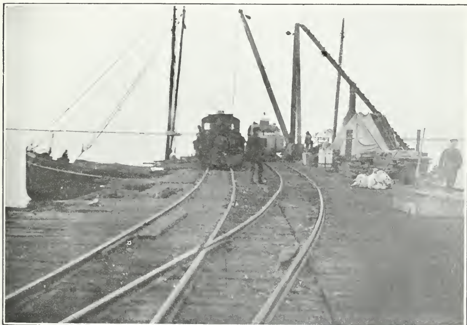
Hudson Bay Railway—Landing materials and supplies at the wharf, Port Nelson.
