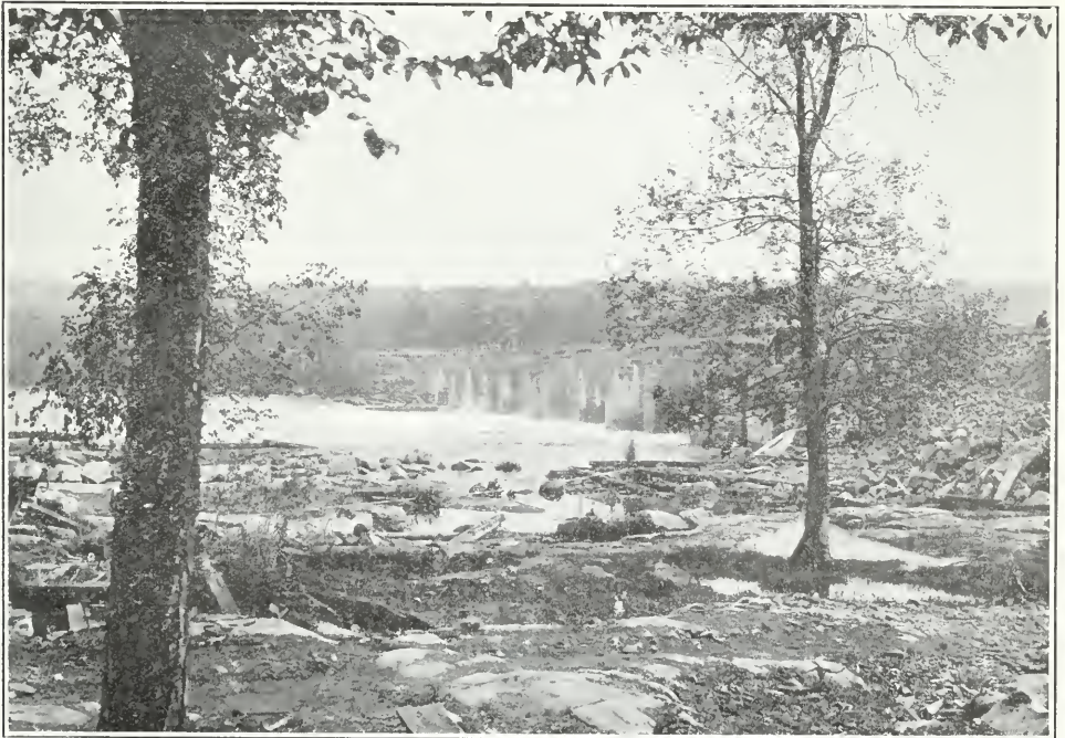
Trent Canal— Down stream view of Burleigh Falls new dam.
