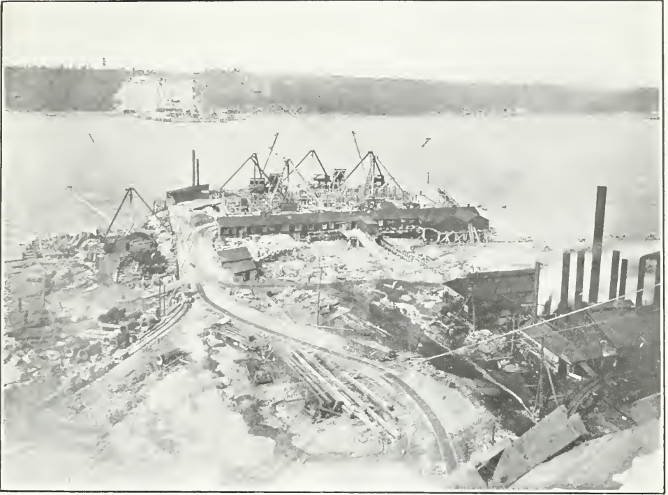
Quebec Bridge—General view of plant on south shore.
