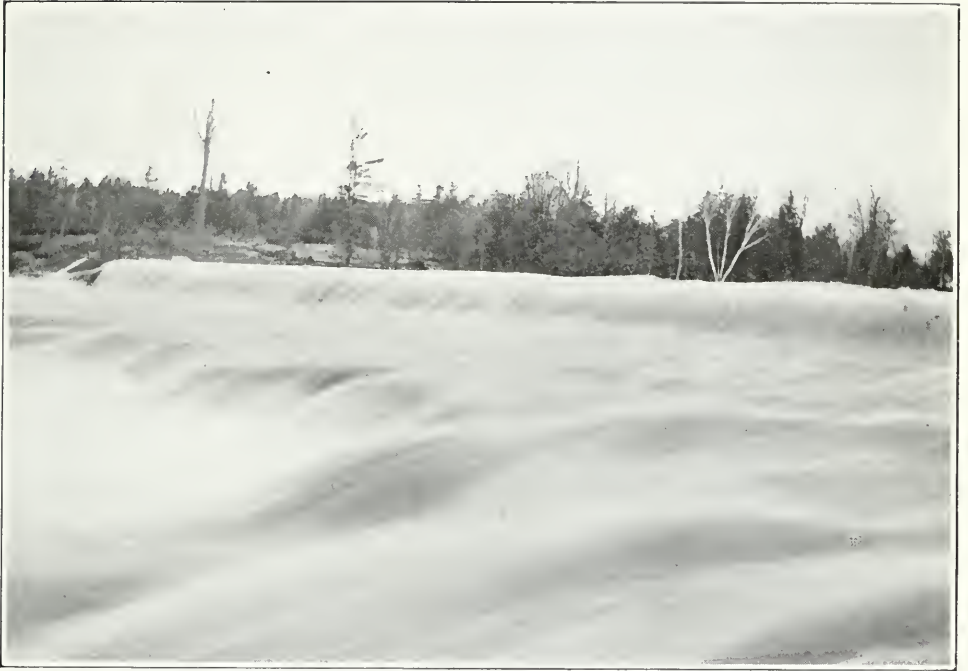
Trent Canal—Crow River Weir. Submerged dam.
