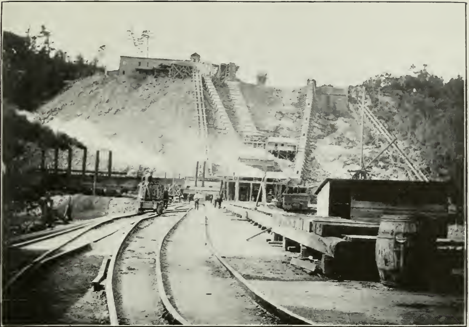
View of north shore showing Boiler, Compressor and Concrete Mining plants. Quebec Bridge in course of construction over River St. Lawrence.
