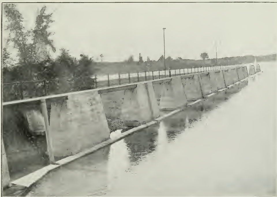
St. Ours Lock, P.Q. Concrete pier below lock (looking west).
