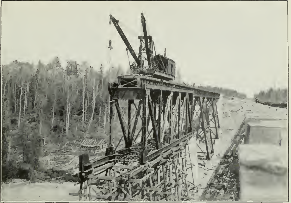
Transcontinental Railway.—Bridge Construction.
