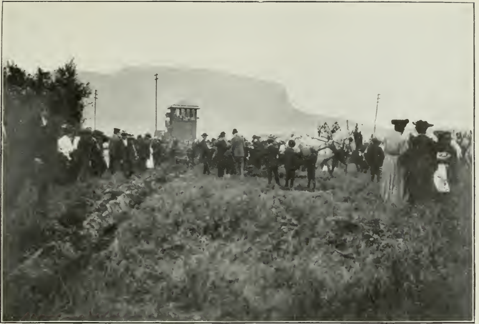
Grand Trunk Pacific Railway.—Turning First Sod at Fort William, Ont
